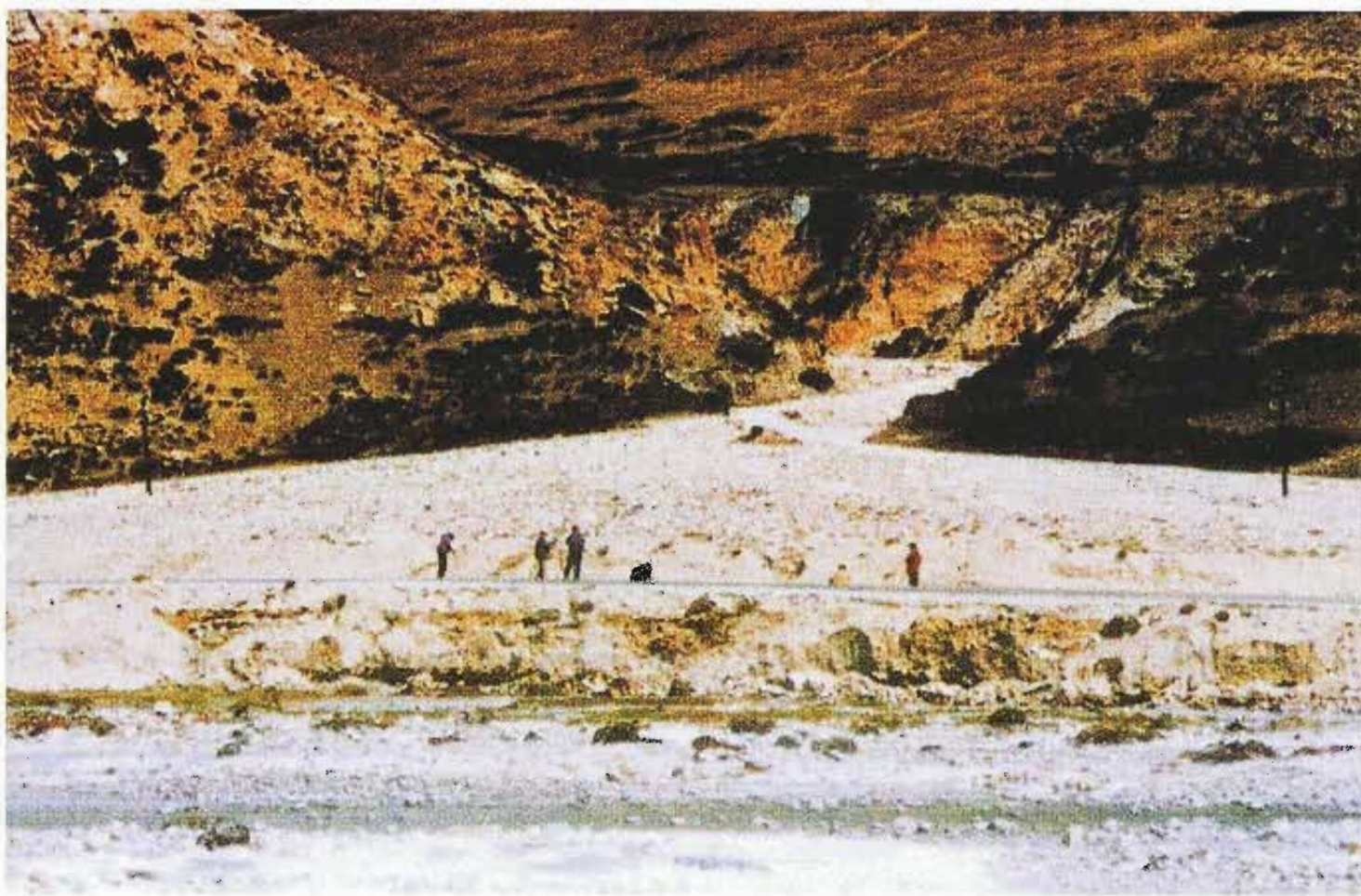
Photo 9-3 The vast debris fan formed by a glacial debris-flow burying the highway (Deng Xiaofeng)
